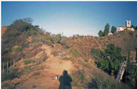
Building site the morning we broke ground, Jan. 1991
