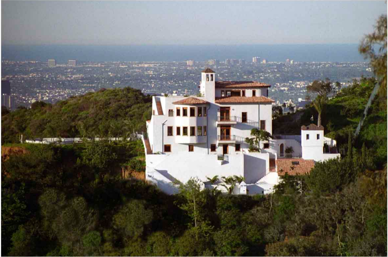
The newly completed Casa de Lila as viewed from another street, looking toward the Pacific Ocean, 1994
